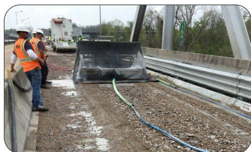
Hydro-Technologies performs hydrodemolition surface prep
