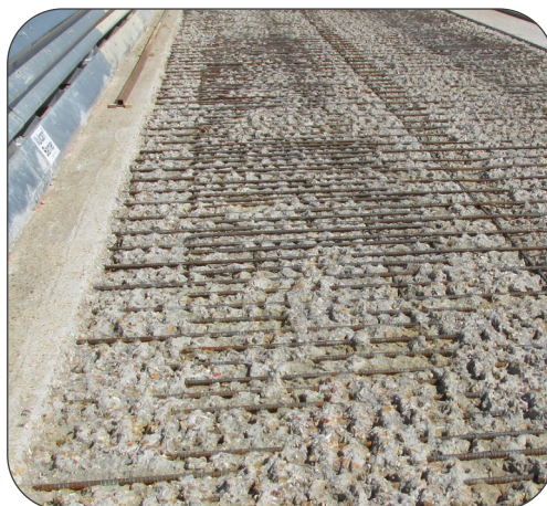
Fast Track method provides a selective removal of concrete
