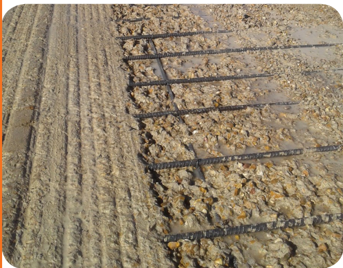
Milling (left), Hydrodemolition surface (right)
