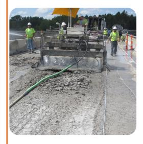
Fast Track Hydrodemolition is a process by which a self-propelled, programmable robot, with a calibrated waterjet, selectively removes concrete. This is done through a single pass of the waterjet. In doing so, not only does it 'selectively remove' all weakened or deteriorated concrete, but it also provides a very roughened and bondable surface for a dense latex modified concrete (LMC) overlay to be monolithically placed.
